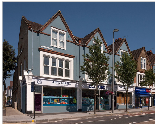
Left: This shop extends across three units, but the fascia sign is broken into sections rather than extending across the whole shop front.
