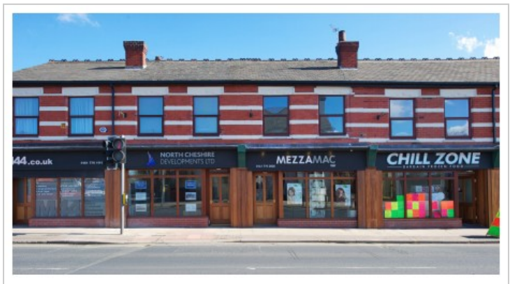
Above: The same shops have been refurbished as a block to ensure a unity of appearance. Individual shop fronts are separated by pilasters whilst signage allows individuality.
